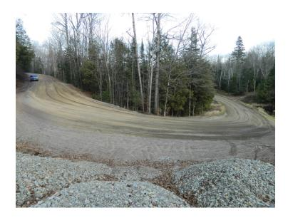
The Old Hastings Road at ?devil's elbow? where Wollaston Township was hoping to reduce the sharpness of the curve on a steep grade.
